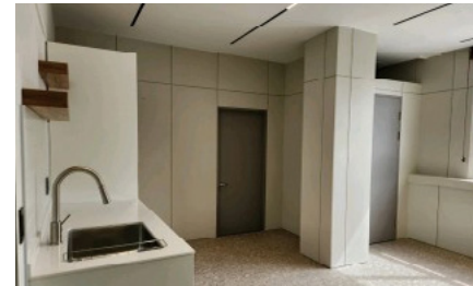
Partially renovated Seogye office (Dec. 2022)
