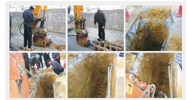
Partial trenchless multi-angle drilling method
