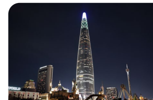
Before Earth Hour lights out
