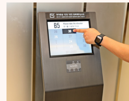
Elevator Destination Panel
