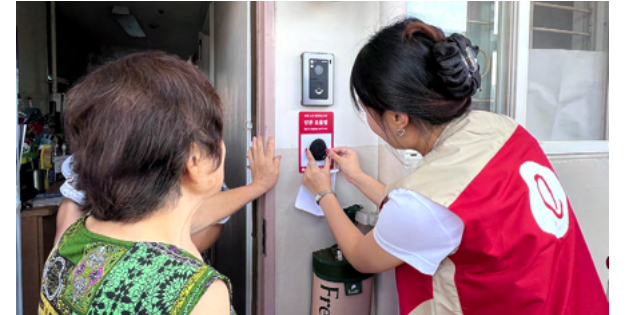
Installation of Wireless Door Lights
