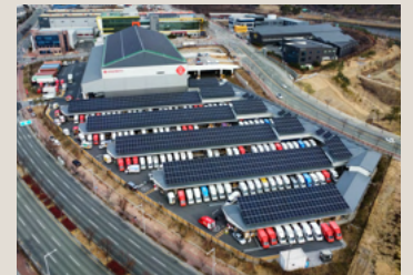
Solar Power Infrastructure at Dongdaegu Sub Terminal
