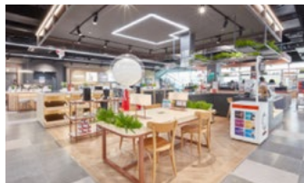
Replacing store LED lights
