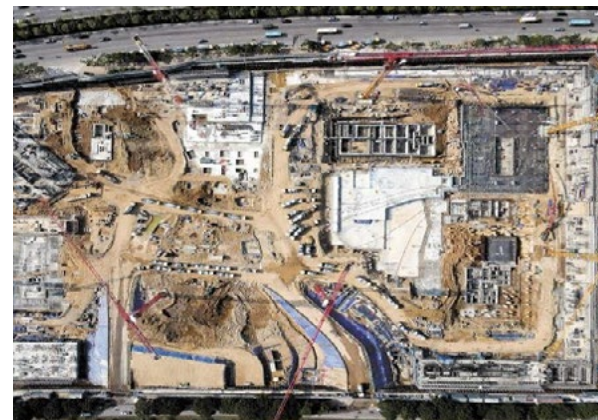
Lotte Mall construction site in Hanoi
