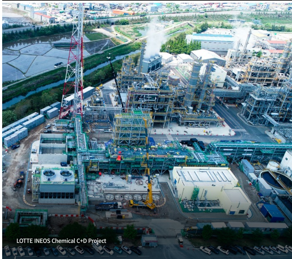
LOTTE GS Chemical G1 Project
