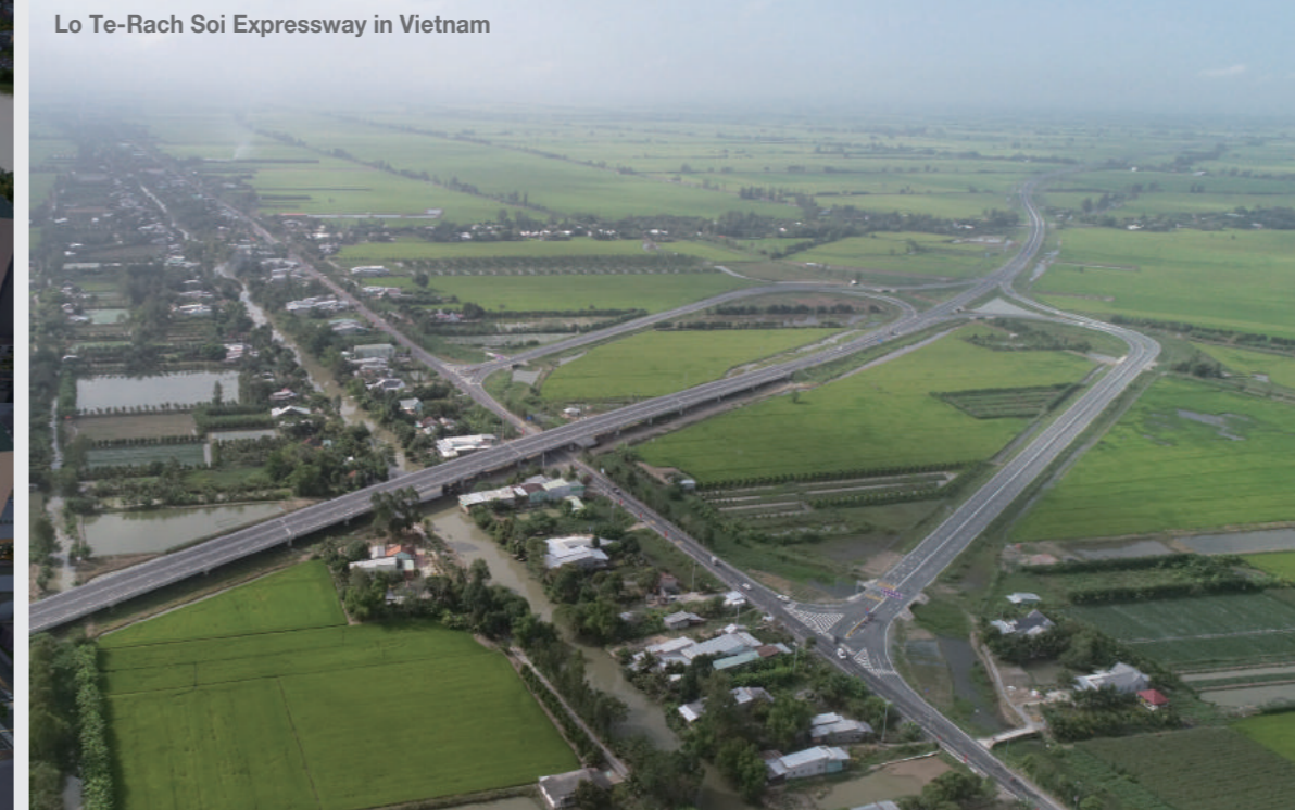
TE-3 Project in Malaysia
