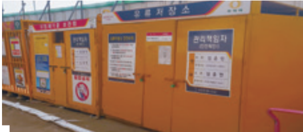
Operating Site-specific Waste Storage Sites
