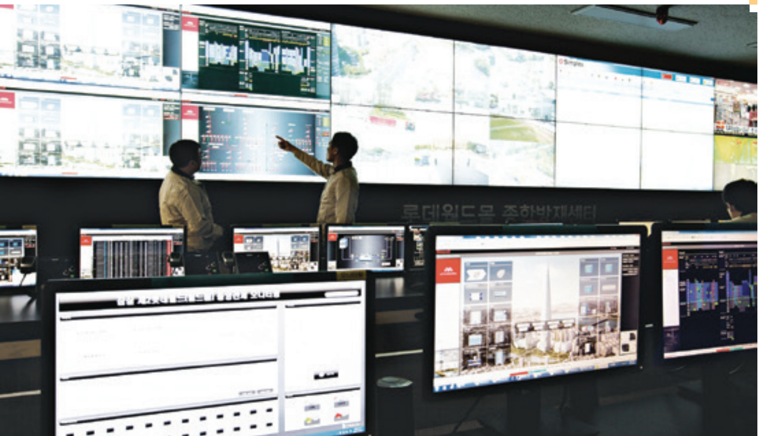
24-hour integrated control center
