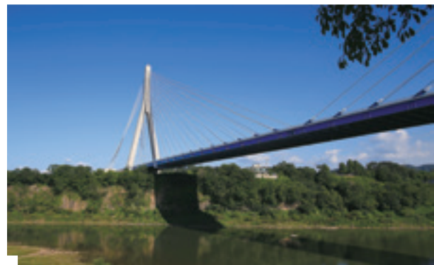
Donggi Bridge, Korea's first long-span, earth-anchored composite cable-stayed bridge
