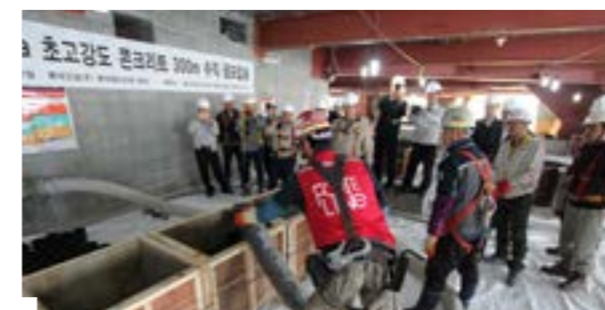
The site where the UHSC vertical pumping was successful for the first time in Korea at 150MPa* * Mega pascal, the strength to support the load of 1.5 tons per unit area of 1cm 2
