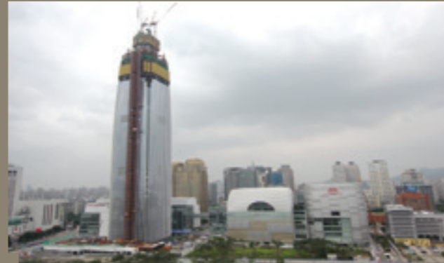
Construction lifts (Hoists)
