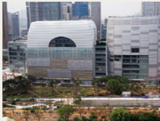
Front view of Lotte World Mall where diverse eco-friendly and new and renewable energy systems are applied
