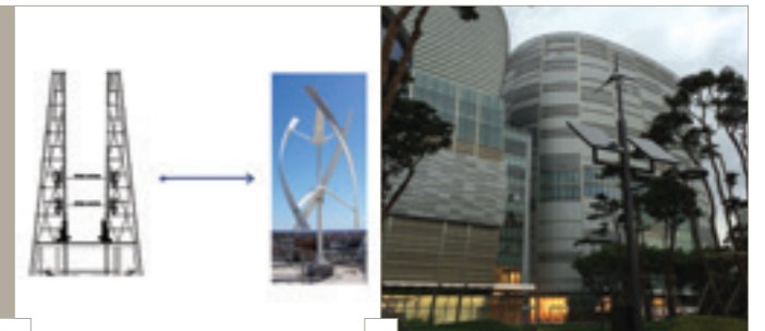
Vertical-axis wind generators
