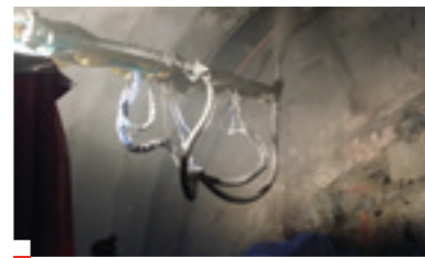
Early Strength-Type Shotcrete
