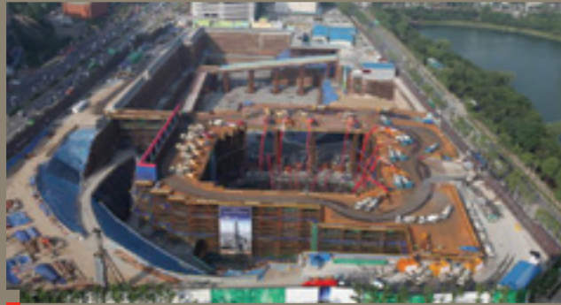
A front side of pumping the MAT foundation
