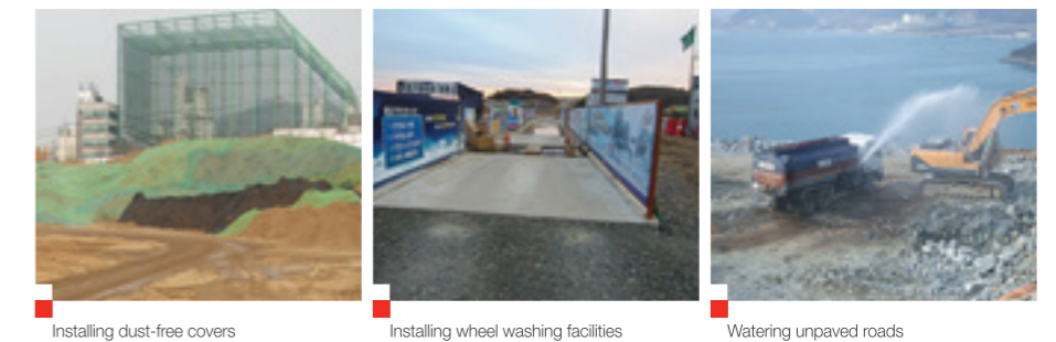
Installing dust-free covers
