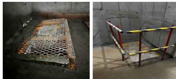
Before and after removing hazardous factors (non-slip measures near staircases)
