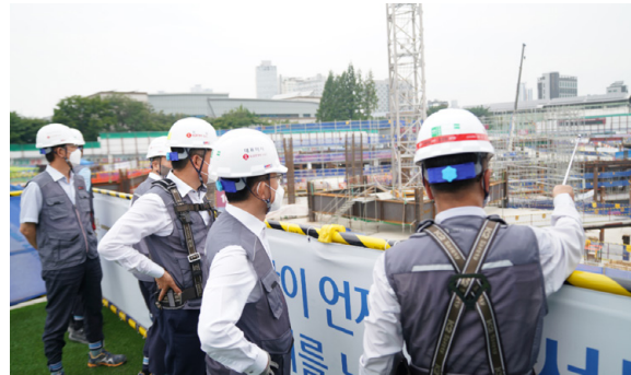
Safety Communication Day (Onsite Inspection)
