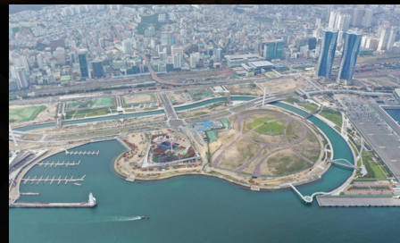
Construction of connecting bridge (Phase 1) of Busan Port (North port) redevelopment project
