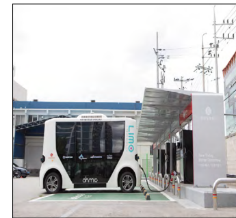
In-house EV charging station
