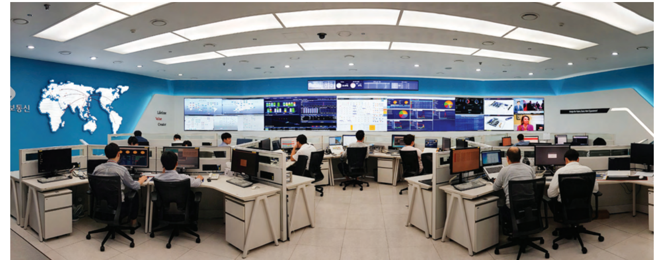
Internal view of data center
