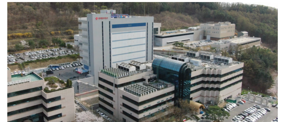
External view of data centers
