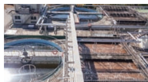
Waste Water Treatment Facility
