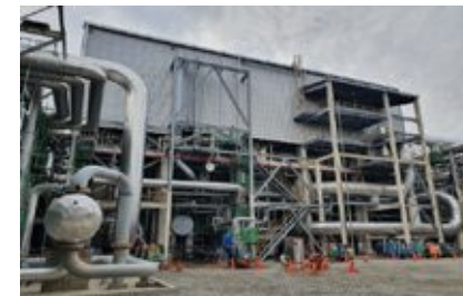
NCC compressor after completion of recovery
