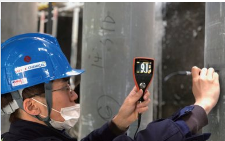
Inspection before operation of NCC plant
