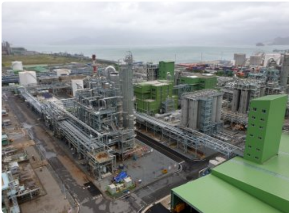
Yeosu PC plant ✓
