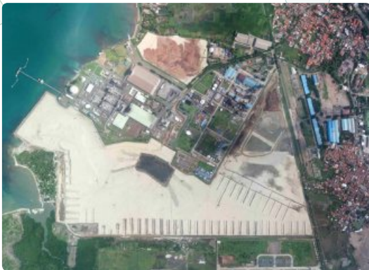
Indonesia petrochemical complex construction site ✓
