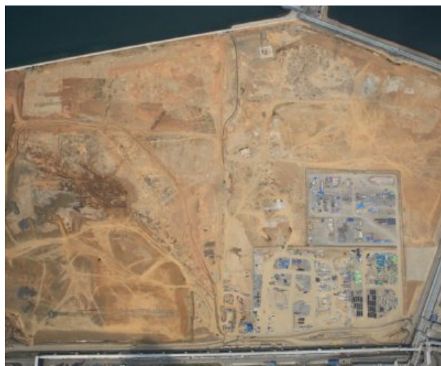
Site Reserved for the Joint Naphtha Cracking Center Project
