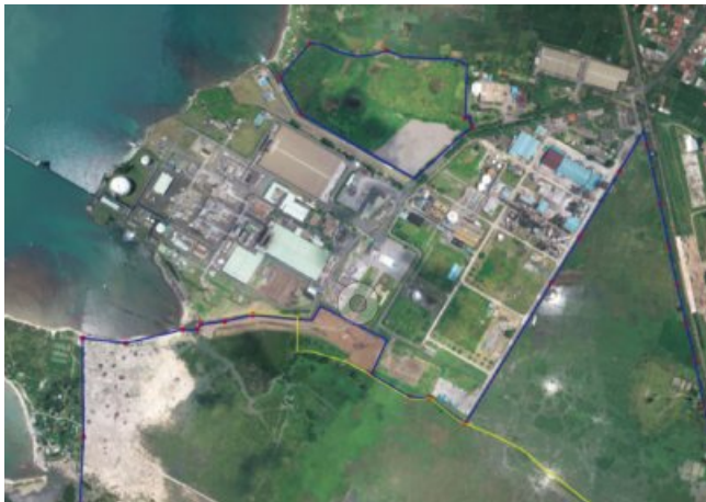
Petrochemical Complex Building Site
