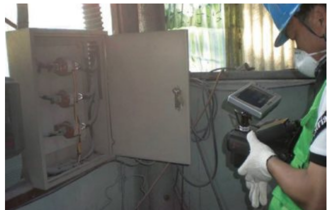
Inspecting an repairing electricity and instruments/machinery
