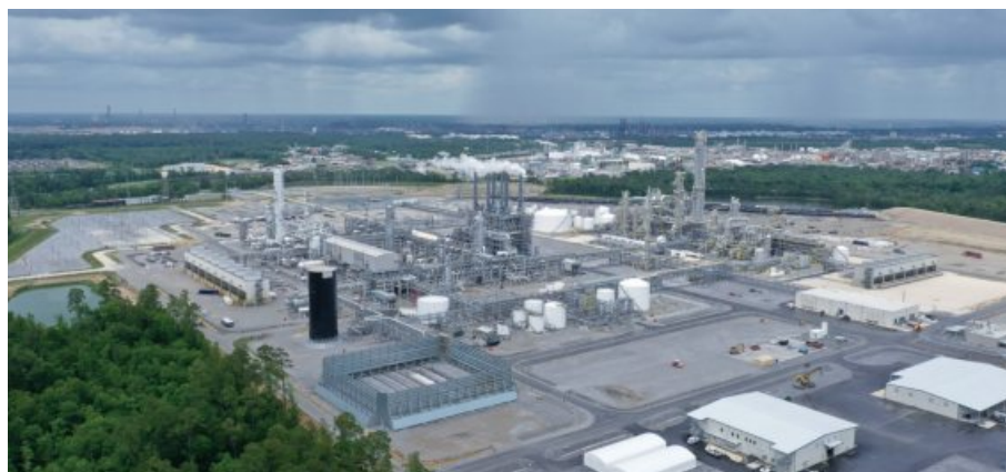
Ethane cracker and ethylene glycol plants under construction in Louisiana, USA
