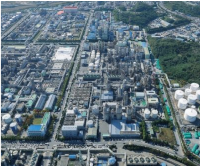
Ulsan Meta-Xylene Plant Expansion
