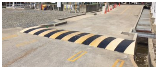
Speed Bump for Tank Lorries Entering and Exiting
