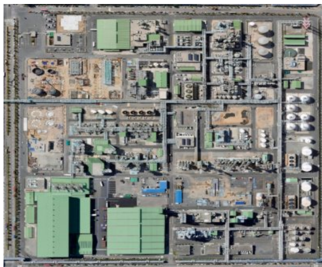
Yeosu PC Plant Expansion
