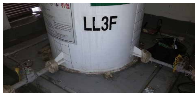
Installation of sulfuric acid leak detector at Daesan Plant tanks
