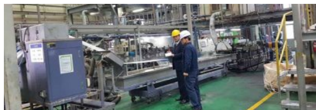
On-site inspection of safety management by subsidiary
