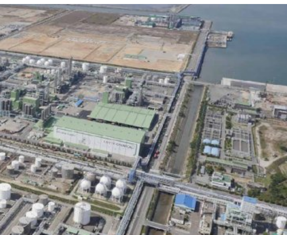
Construction of Daegu Water Treatment Membrane Plant
