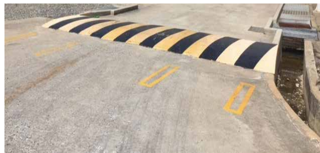
Flow prevention bump for tank lorry
