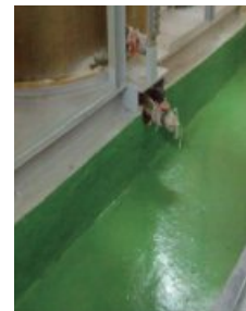
Daesan Plant: floor coating with impermeable materials
