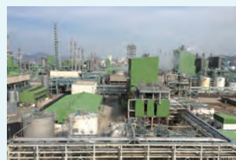
Commercial Production of PE Catalyst in Yeosu National Industrial Complex
