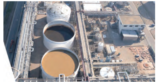
Installation of Wastewater Transfer Facilities
