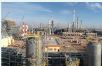
Petrochemical Plant in Uzbekistan
