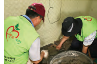
Providing Additional Services to Fix the House
