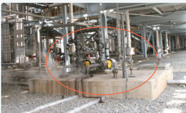
Recycling blow-down water in steam drum of naphtha cracking furnace for the use of coolant(Apr 2002, 240 T/D)
